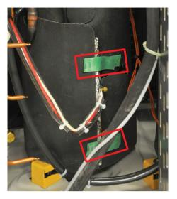
7. Check that crankcase heater(s) is (are) heating when powered. If not, the crankcase heater(s) must be replaced. Refer to "Replacing a crankcase heater E1HC, E2HC" on page 176.
