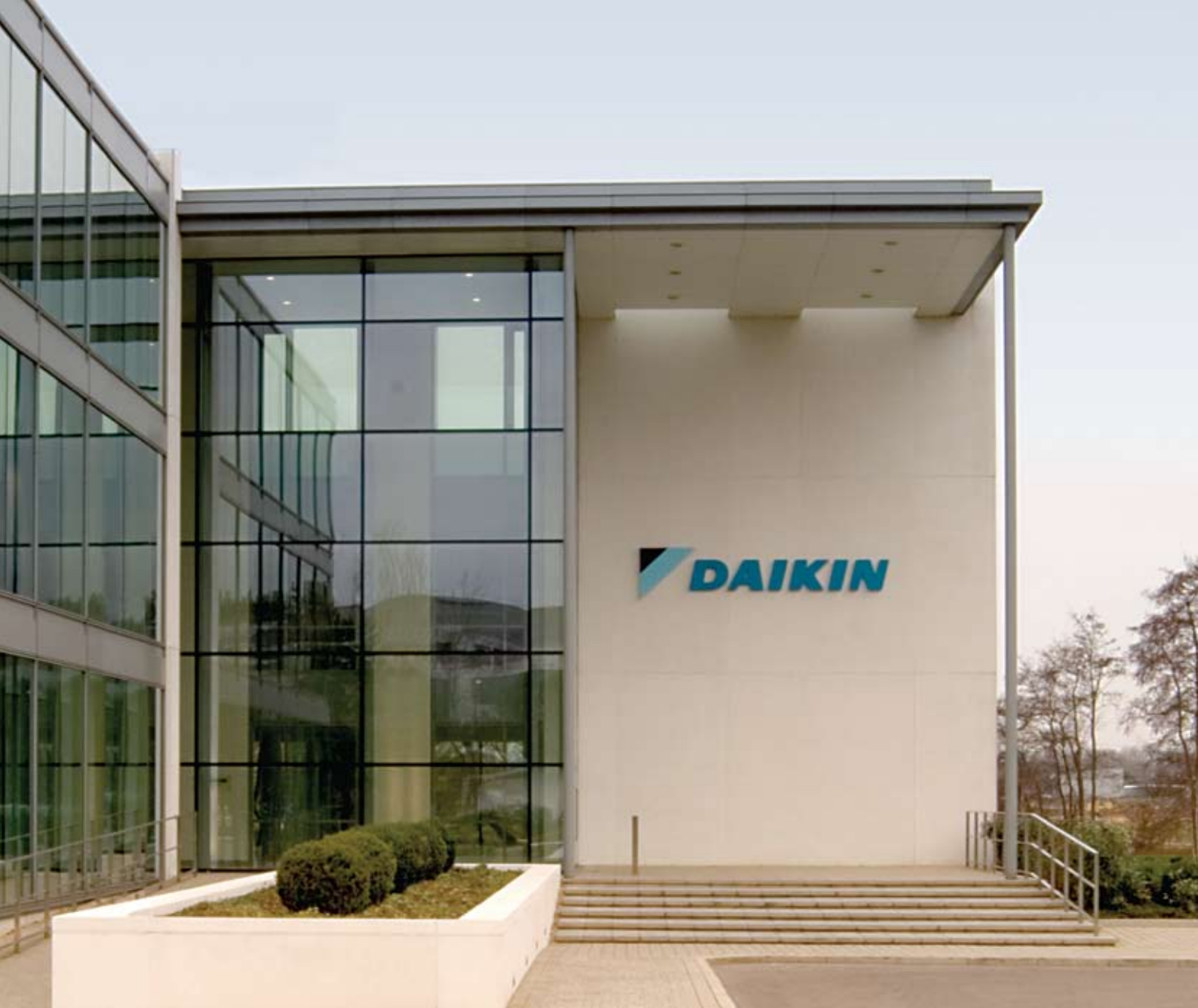
Daikin Airconditioning UK Ltd, Weybridge Head Office
