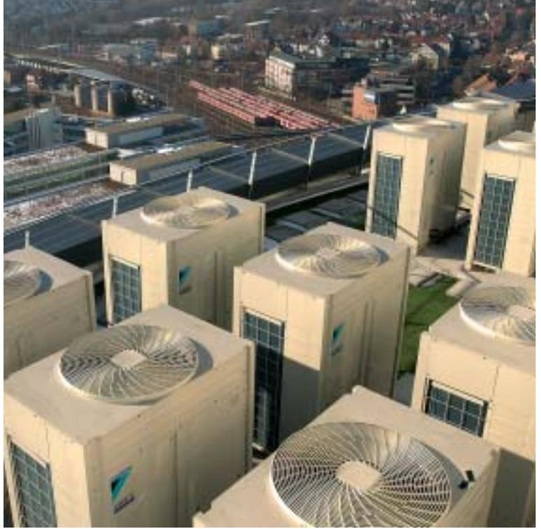
Many features and installation benefits are incorporated in VRV II. Its operating range for example 8hp to 48hp in 2hp increment steps (21 system combinations), is wider than any of its contemporaries. Furthermore, its ability to run no less than 40 indoor units in heat recovery format cannot at present be matched by other comparable systems.
